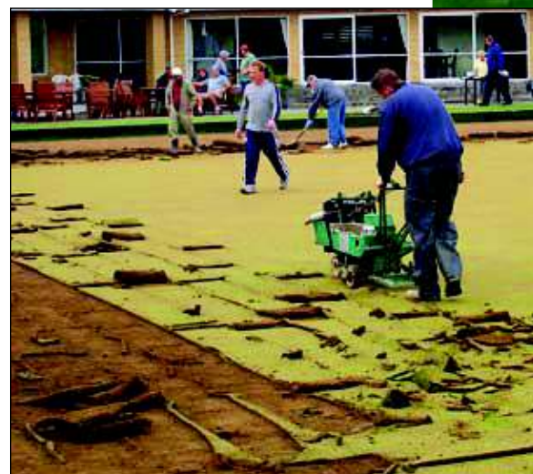
Resurfacing – one option for providing a uniform cover.
